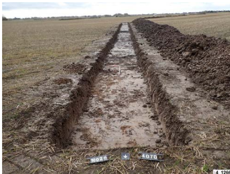
Plate 408: Field D-3-05 Trench 4070 facing south (scale: 2 x 1m)
