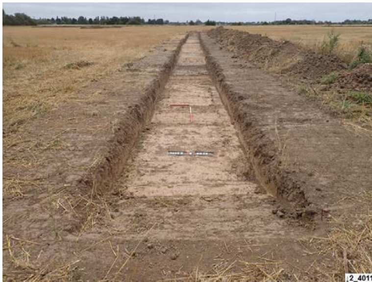
Plate 470: Field D-6 Trench 4037 facing south (scale: 2 x 1m)
