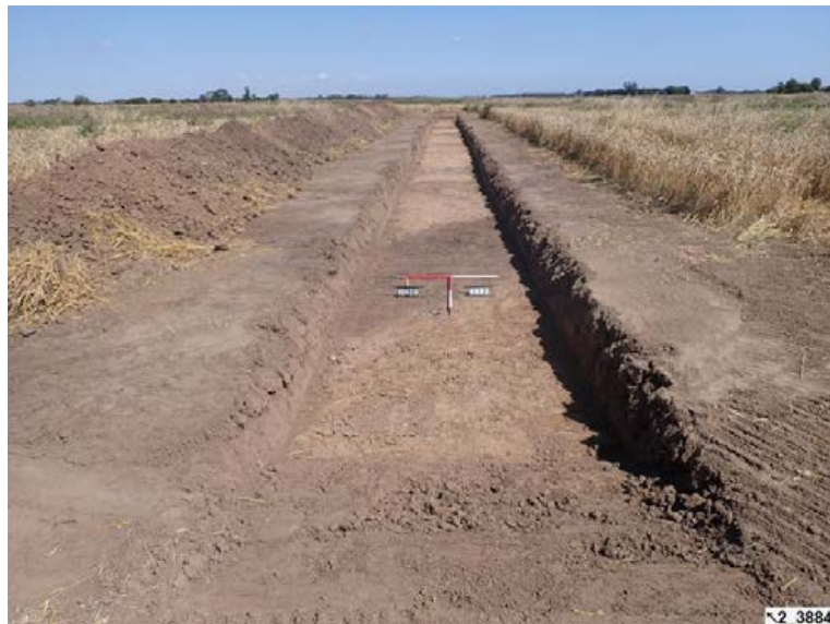
Plate 462: Field D-6 Trench 4032 facing north-east (scale: 2 x 1m)
